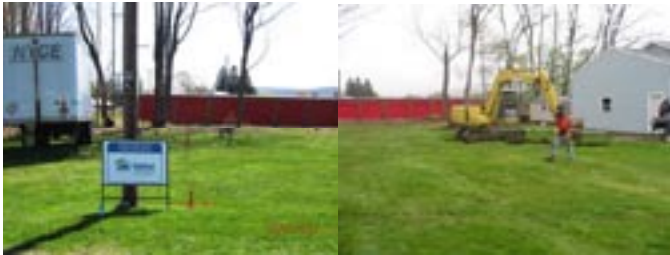
April 24 – 28: ground has thawed and excavation begins
