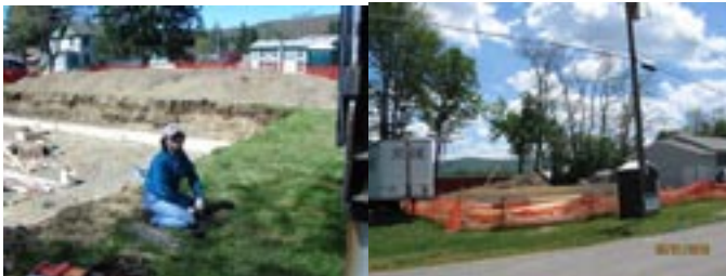
April 29: Barb Dauria digs in, May 31: lot is staked
