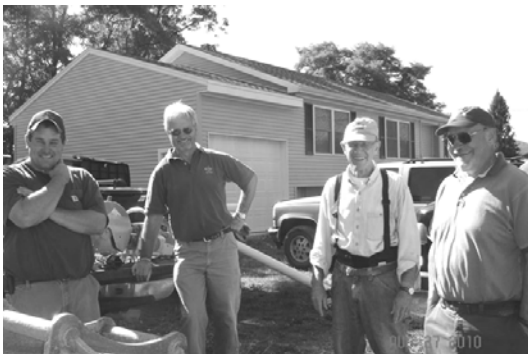
(L-R) Mike Saggese and Paul Biesler, of Seward Sand and Gravel, shown with HFHOCers Bruce Downie and Mike Donahue. Mike and Paul donated a day of labor on our water and sewer excavation.
